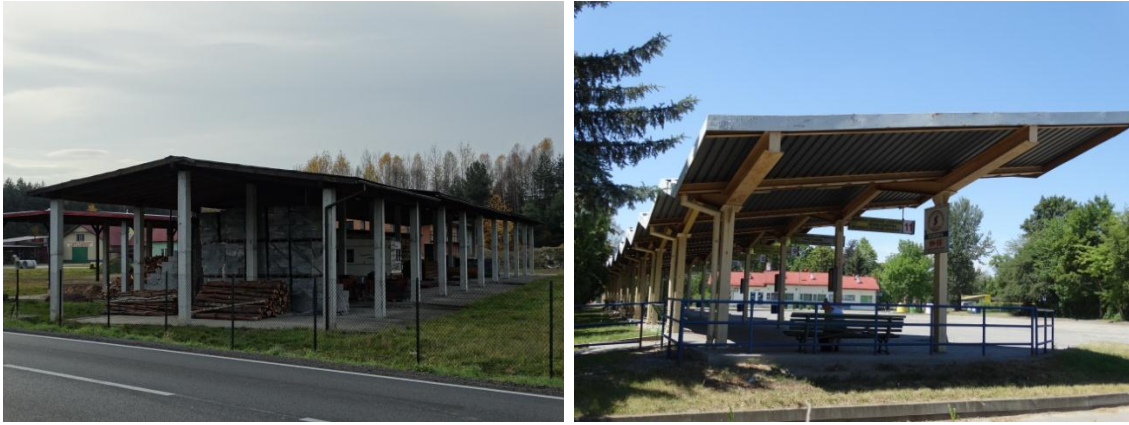
Fig. 5. Shelter - a special kind of building by PKOB (Foto: M. Buško)
