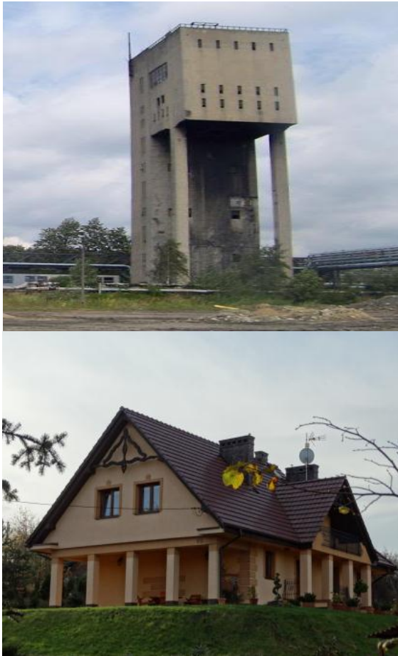
Fig. 3. Buildings in which the edges of the walls based on the pillars are not their extension (Foto: M. Buško).
