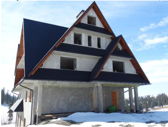
Fig. 4. The edges of the walls based on the pillars are not their extension (Foto: M. Buško)
