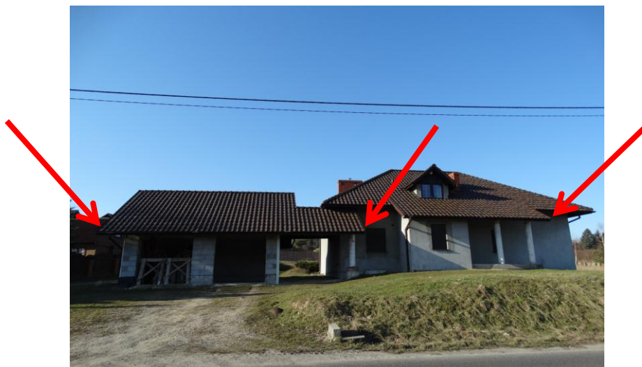
Fig. 7. The building with a roof based on the pillars (Foto: M. Buško)
